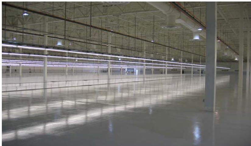
Finished Floor 2-Roll Coat Applications
